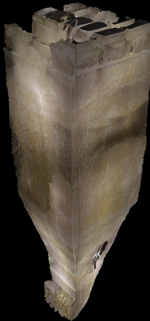
Point cloud generated photogrammetrically from inspection video
